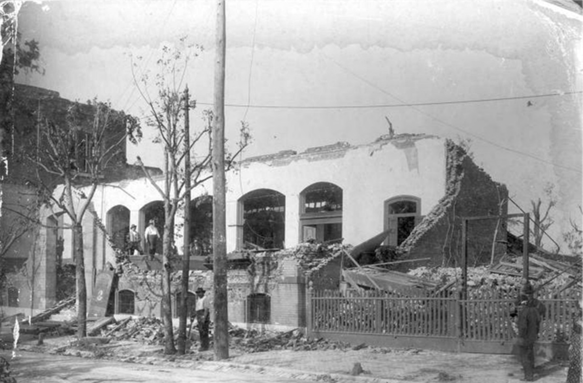
1726 S 18 th St (saloon/brewery) (presently I-44 EB off-ramp to Lafayette Ave) Looking East
