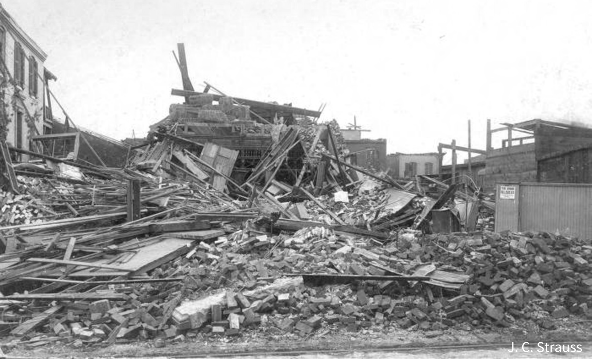
Ruins of Fire Station No. 7 1304 S. 18 th St Looking East
