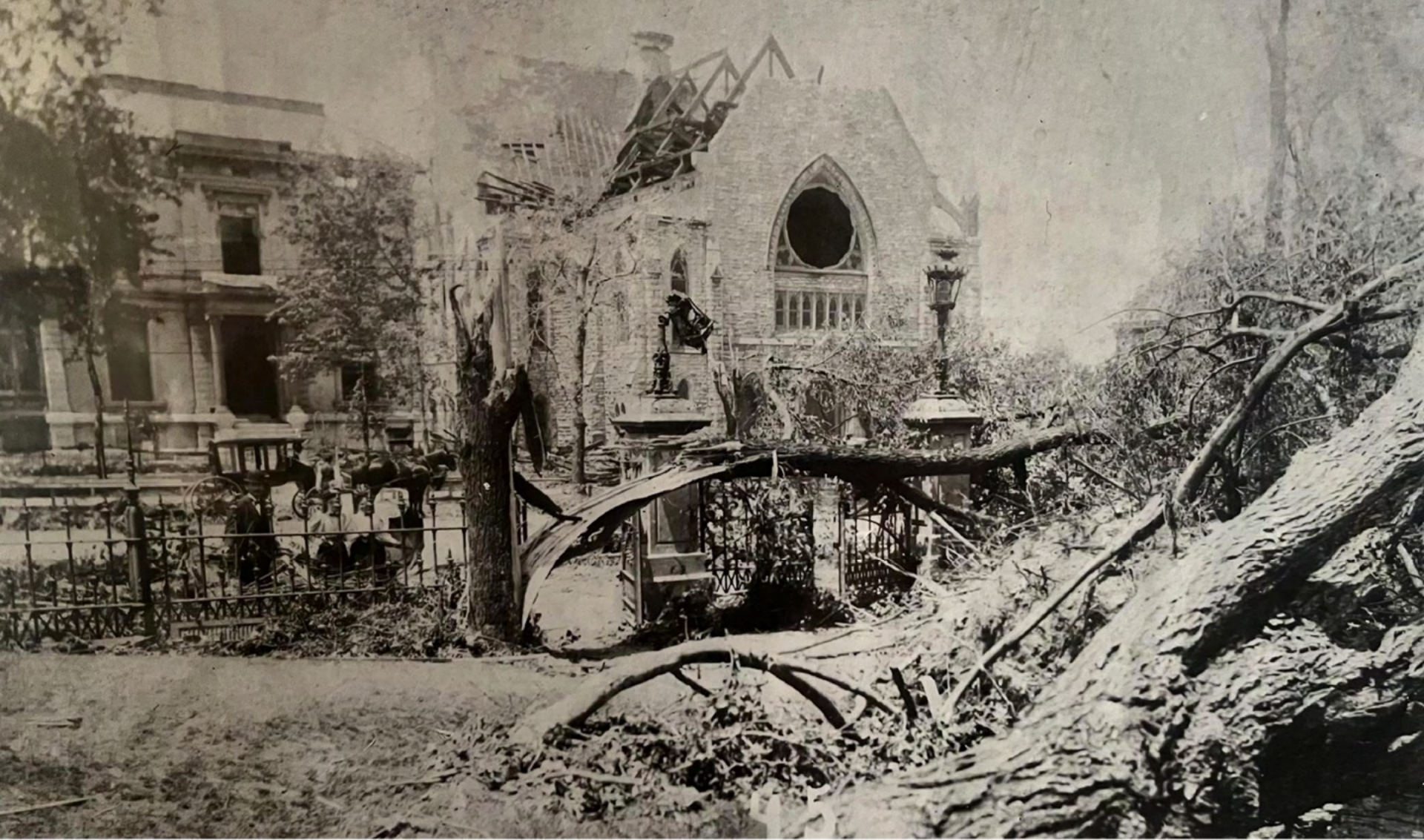
1515 Missouri Ave & Lafayette Park Presbyterian Church Looking West
