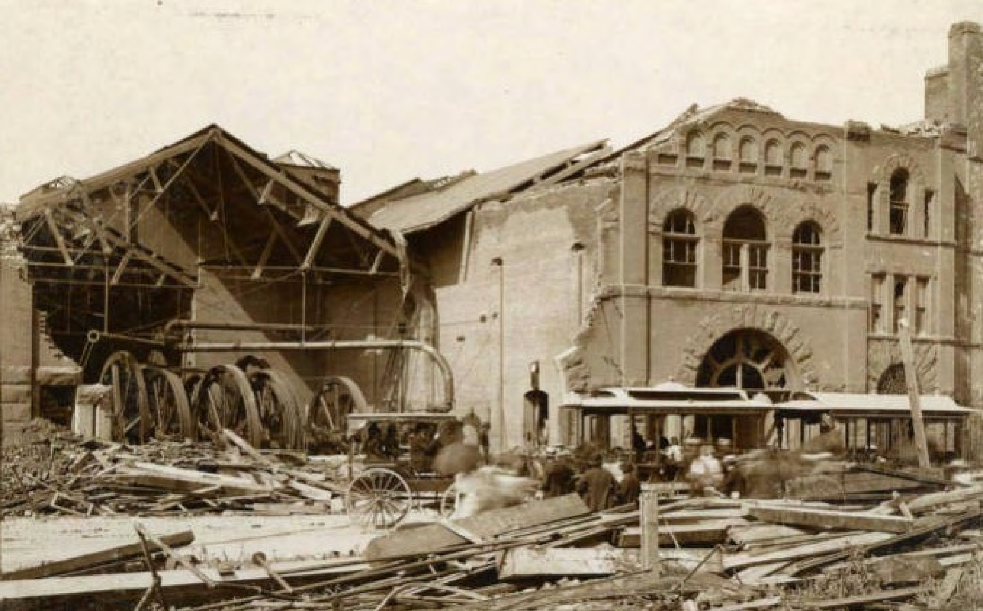
People's Railway Co. Powerhouse At Park Ave & S. 18 th St (present site of Fountain View on Park Condos)
